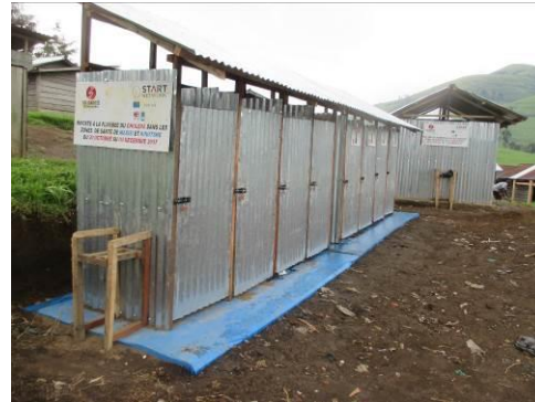
Photograph 2. WEDC - Latrines completed in Rubaya
