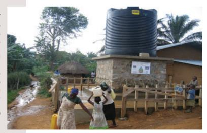
> One of the 22 public tap stands constructed in Kalemie in the DRC, equipped with a reservoir of 10m3 and a row of 10 taps
