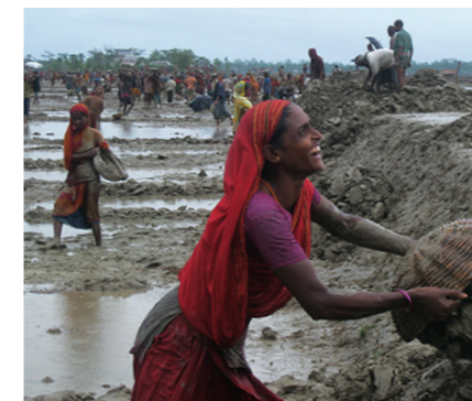
Building a dyke in Bangladesh.
