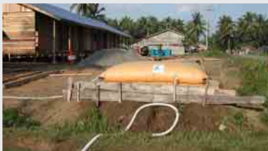
A flexible drinking water tank set up by SOLIDARITÉS and Aquassistance in Sumatra (Indonesia)
